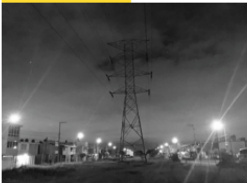
Torre A 10 pm.
