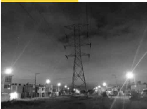
Torre A 10 pm.
